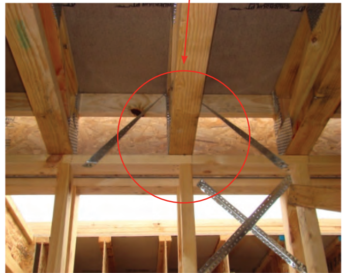
Additional bracing
