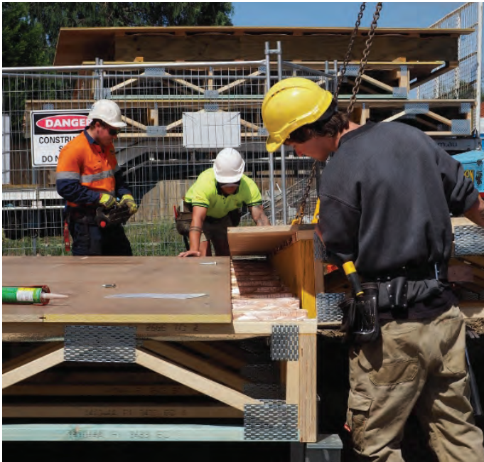
Ensure neat fit of subsequent cassettes
