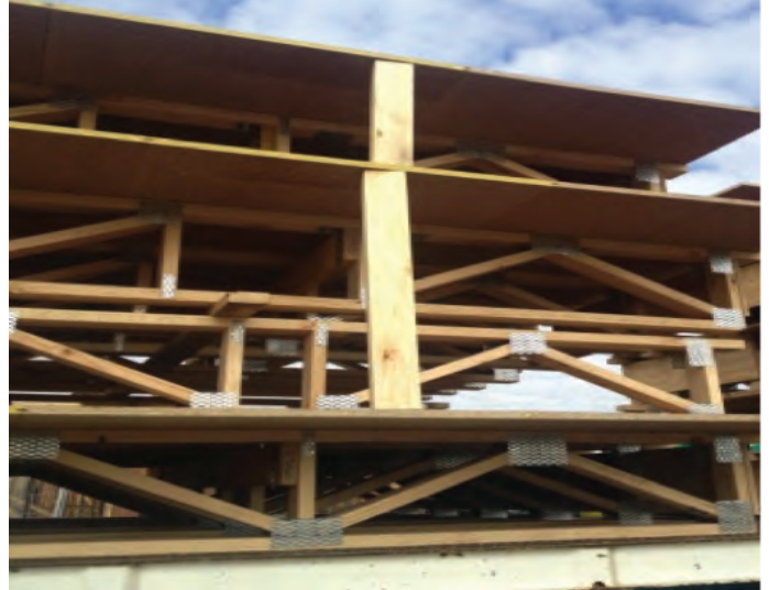
End block to avoid floor sheet damage
