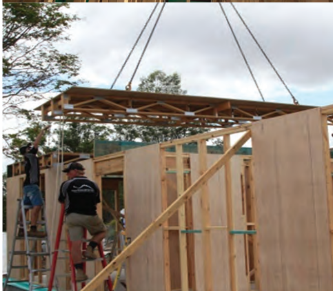
Upper storey cassette installation
