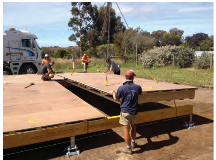
Ground floor cassette installation
