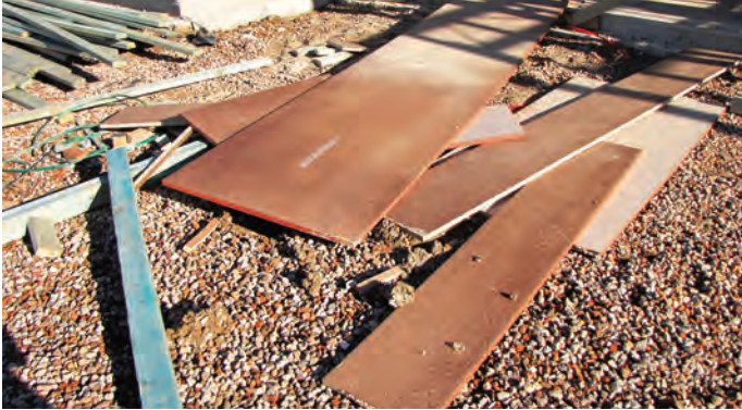
Onsite wastage for floor sheeting
