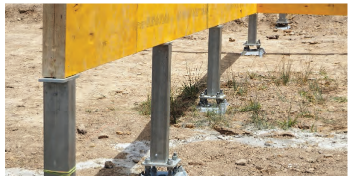
Align bearers and fix to post caps
